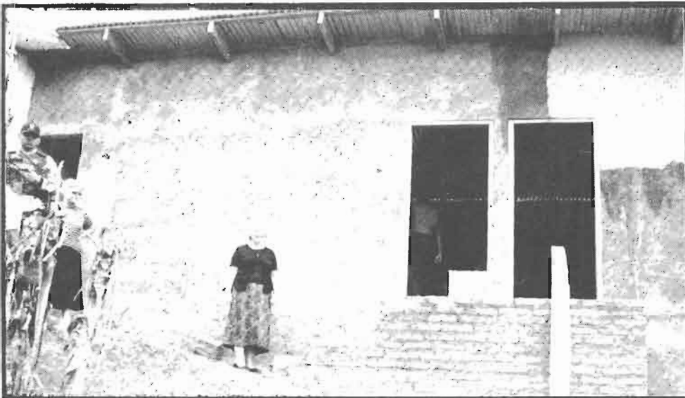
Construction of Sunday School Rooms and Pastorium in Los Planes, Duyure, Honduras
