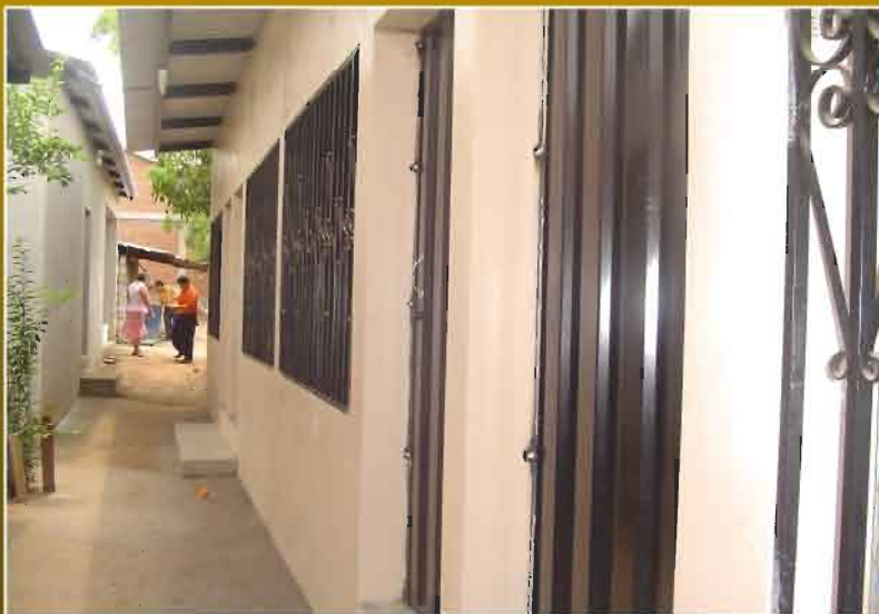
New S.S. Rooms and Pastorium in Maranatha Baptist Church, our third church in Choulteca
