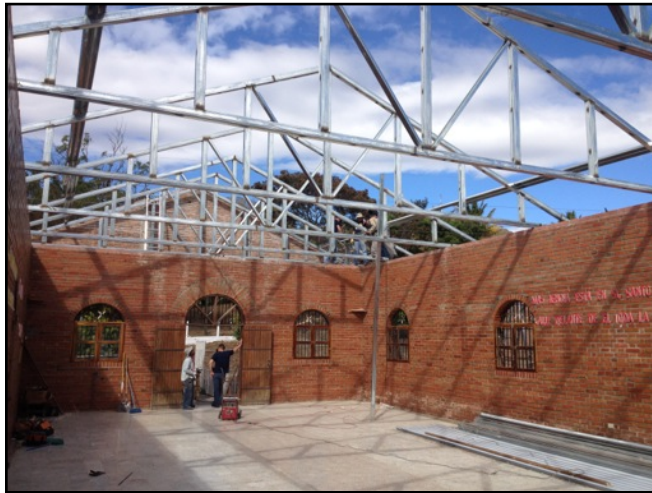
Roof under construction of the church in San Francisco, Honduras
