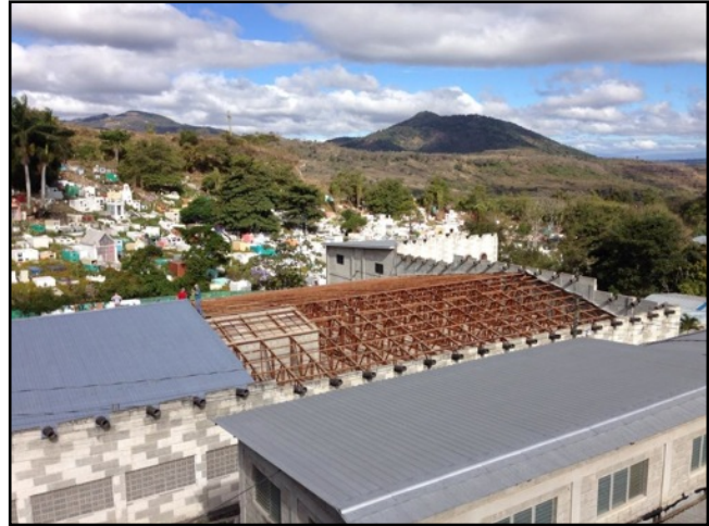
New roof being put on of Good Samaritan Elementary School
